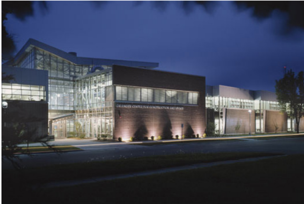
FERRIS STATE GRANGER BUILDING
